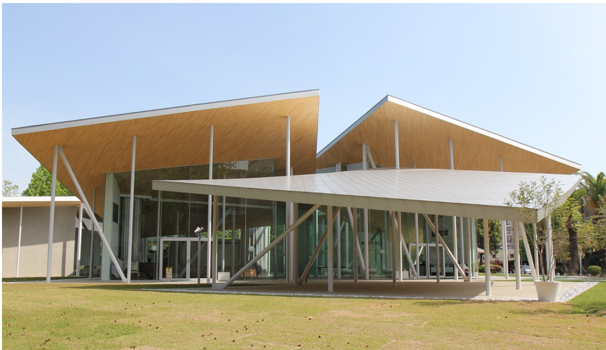
「Junko Fukutake Hall」 Kazuyo Sejima + Ryue Nishizawa / SANAA Okayama University (Shikata Campus, Okayama City) http://www.okayama-u.ac.jp/eng/access_maps/index.html
