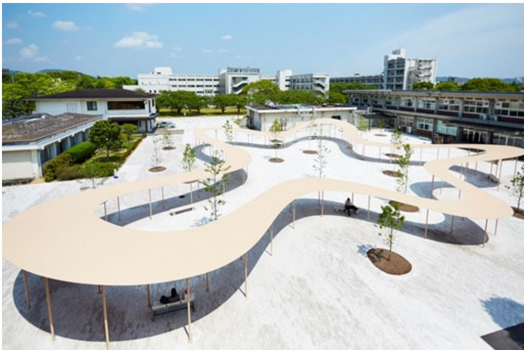
「Pergola」 Kazuyo Sejima + Ryue Nishizawa / SANAA Okayama University (Tsushima Campus, Okayama City) http://www.okayama-u.ac.jp/eng/access_maps/Tsushima_Campus.html
